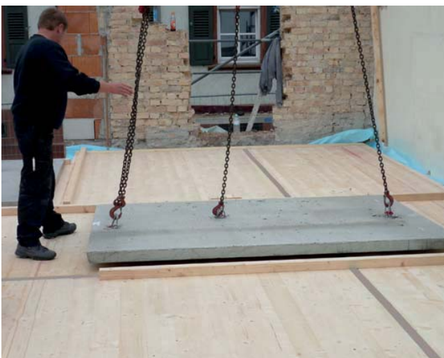
Installing pre-fabricated slabs with FP connectors on board stack elements
